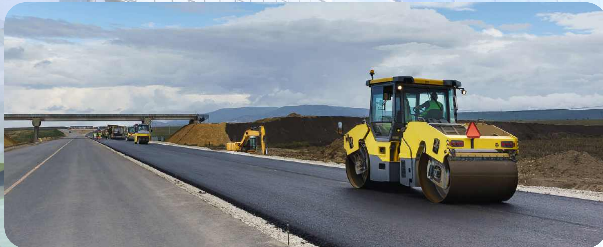
Road Construction | Kegoz Group
